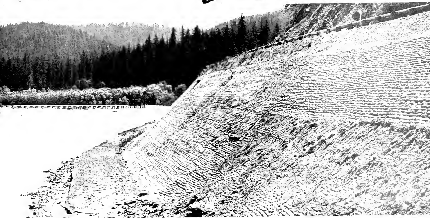
Angular timber deflectors protecting banks and Redwood Tree groups shown above. At bottom riprap section that successfully withstood flood currents.
